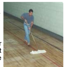
Tacking floor with cotton towels and push broom.
