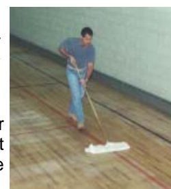
Tacking floor with cotton towels and push broom.
