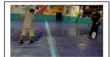
Application of Crimp Coat with sprayer and microfiber mop.
