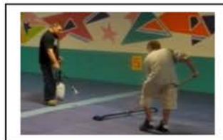
Application of Crimp Coat with sprayer and microfiber mop.
